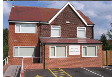
The Lanes Medical Centre
